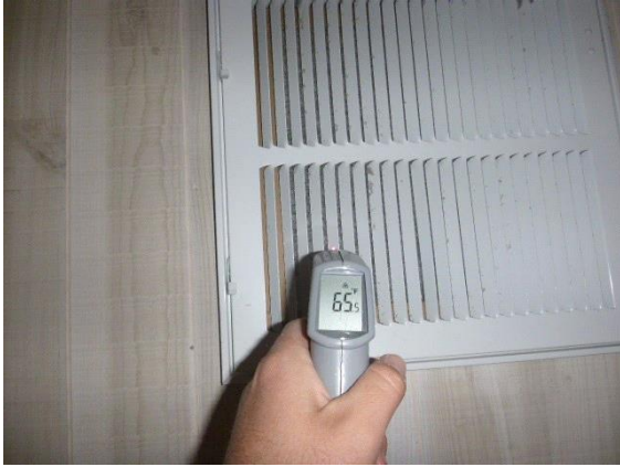
Heating: View of 2nd floor return air temperature using a digital thermometer in the heating mode
