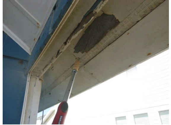
Exterior Surface: View of one location of soft deteriorated wood soffit and fascia
