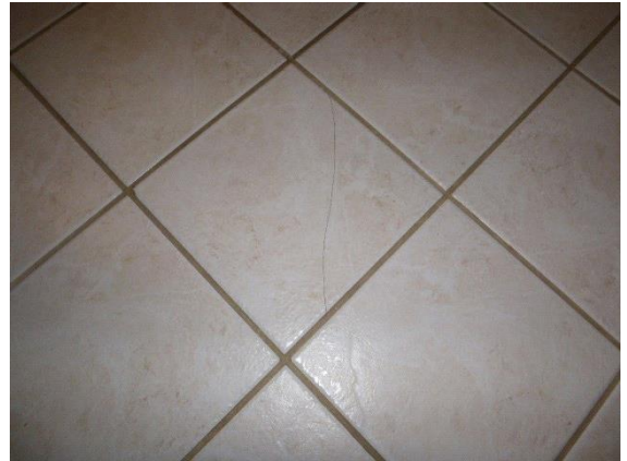
Bathroom #3 - 2nd Floor : View of one location of cracked bathroom ceramic floor tiles
