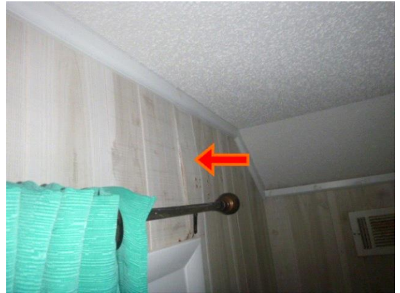
Bedroom #5 - 2nd Floor - Rear : View of one location of buckling in wall paneling
