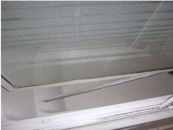
Bathroom #4 -1st Floor Left: View of damaged shower enclosure door
