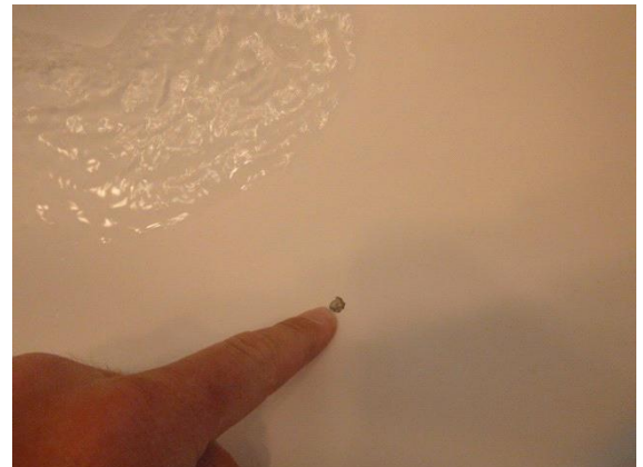
Bathroom #2 - 1st Floor Right: View of hole in bathroom sink
