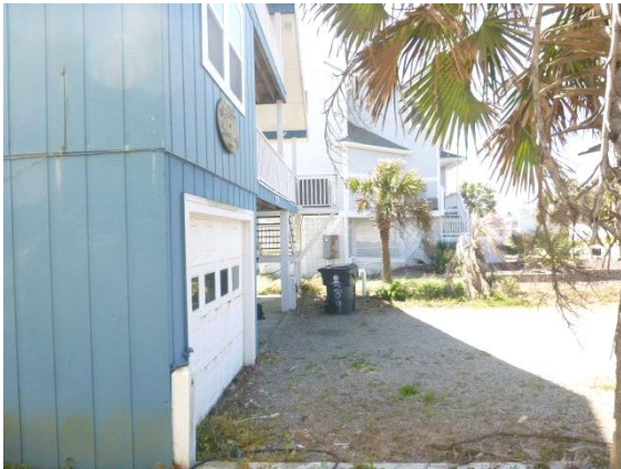
Grading / Drainage: View of front property
