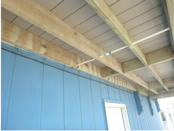
Decks - 1st Floor - Rear : View showing the deck ledger board not bolted to the house, and no joist hangers or ledger strips present
