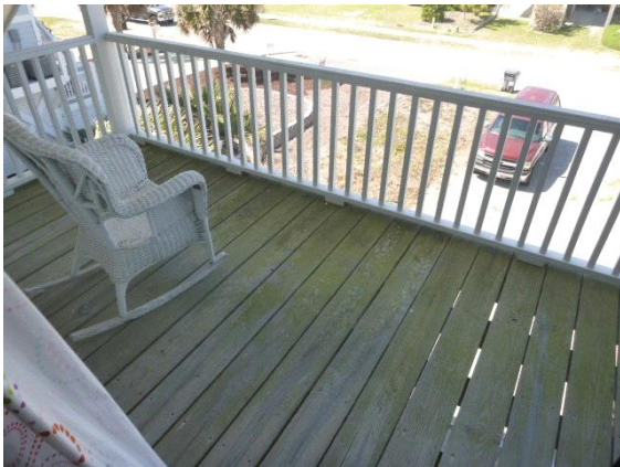
Decks - 2nd Floor - Front : Overall view of front 2nd floor wood deck
