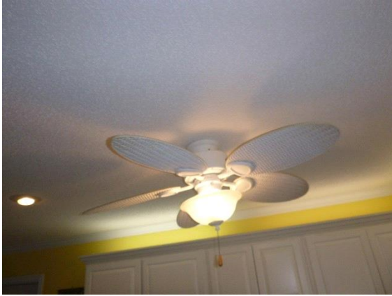
Kitchen: View of ceiling fan that did not operate
