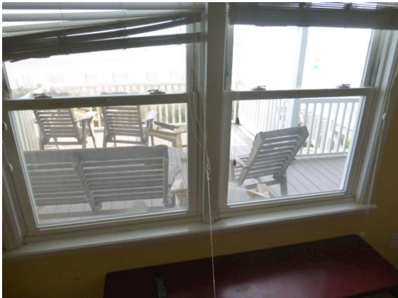
Living Room: View of defective living room windows
