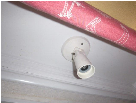
Kitchen: View of bulb missing from kitchen fixture
