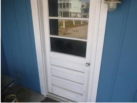
Carport/Under House: View of one location of ground floor entry doors that could not be accessed with key
