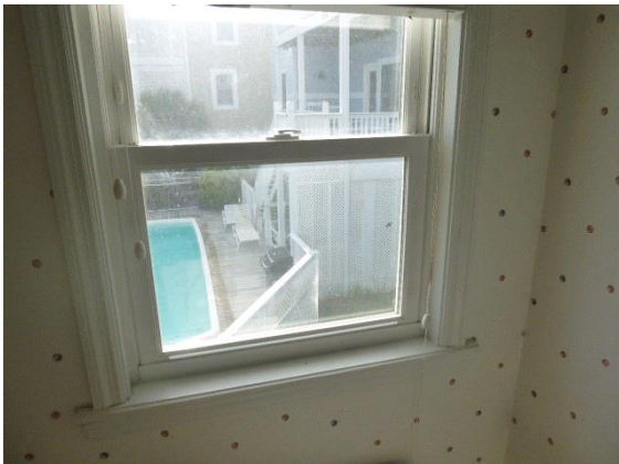
Bathroom #2 - 1st Floor Right: View of window that slams shut when operating
