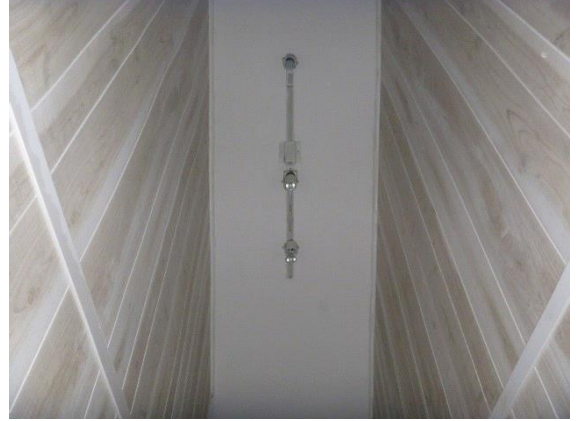
Stairs / Railings: View of defective light fixture located above the stairwell leading up to the 2nd floor
