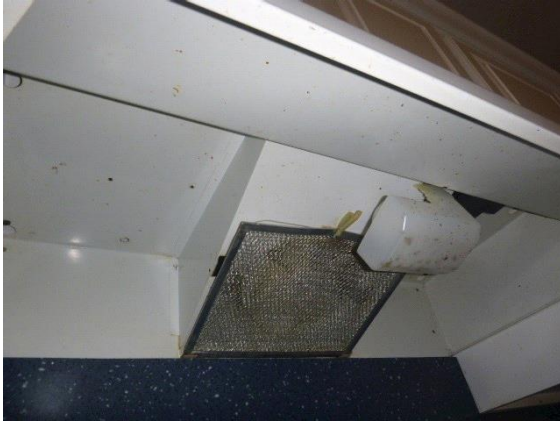
Kitchen: View of exhaust fan that made excessive noise when operating
