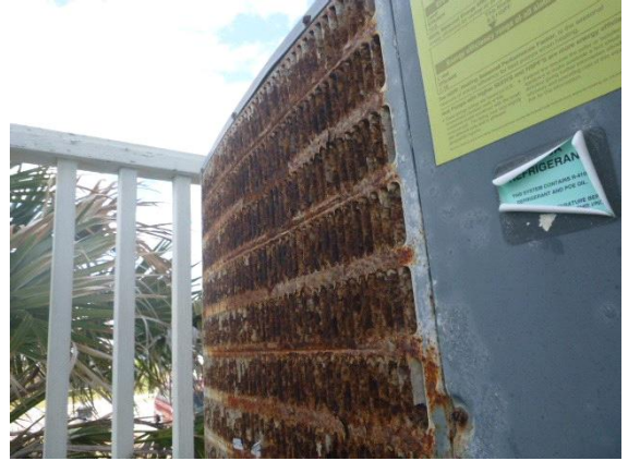
Heating: View of one location of excessive corrosion present on the outside condenser unit
