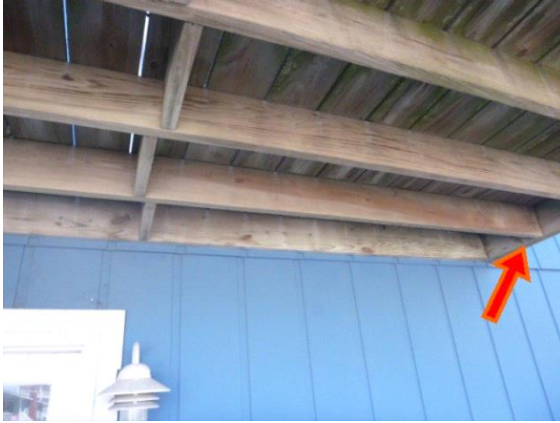
Decks - 2nd Floor - Front : View of missing joist hangers or ledger strips located at the ends of the floor joists
