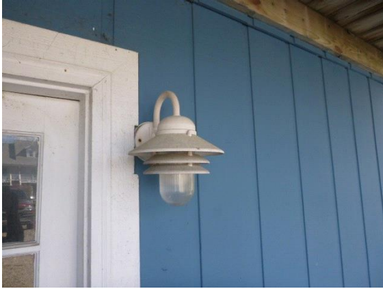
Exterior Surface: View of one location of defective exterior light fixtures
