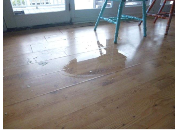
Living Room: View of water noted on living room floor at the time of inspection
