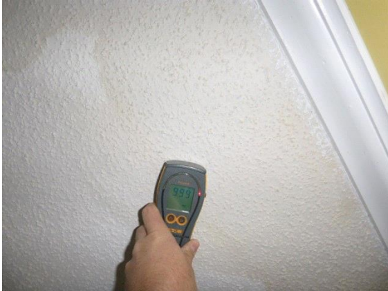
Living Room: View of moisture meter indicating ceiling stains are wet
