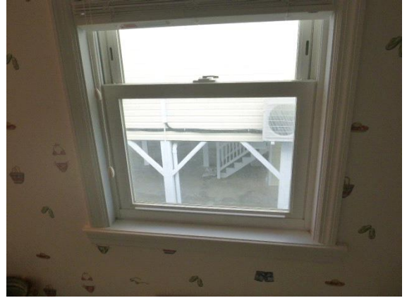
Bathroom #4 -1st Floor Left: View of window that slams shut when operating
