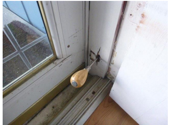
Exterior Doors: View of one location of soft wood present at front entry door
