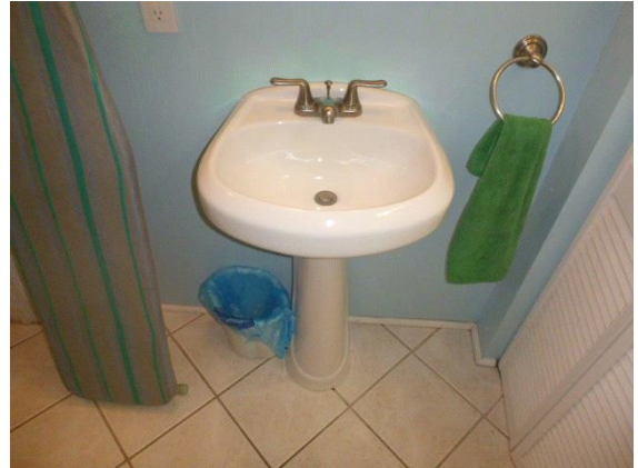
Bathroom #1 -1st Floor Middle : View of pedestal sink loose from wall
