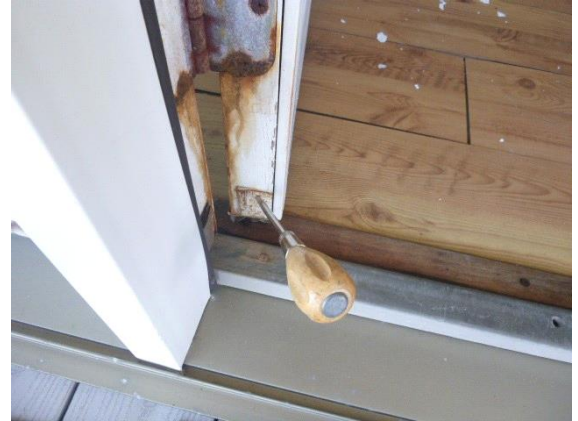
Exterior Doors: View of one location of soft wood present at rear entry door
