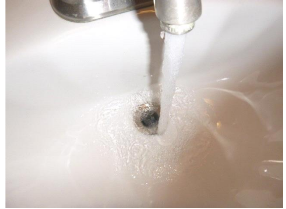
Bathroom #3 - 2nd Floor : View of missing stopper located in the bathroom sink
