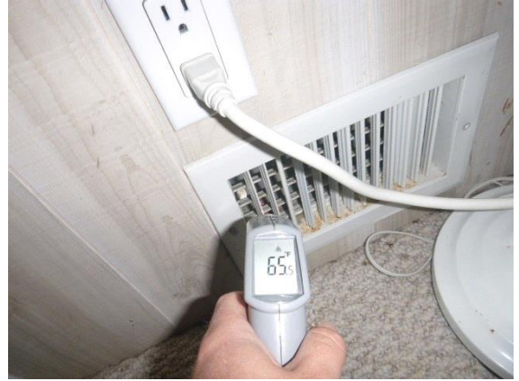
Heating: View of 2nd floor supply air temperature using a digital thermometer in the heating mode
