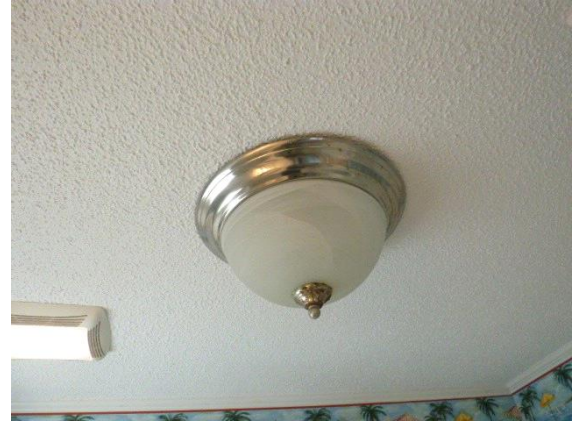
Bathroom #2 - 1st Floor Right: View showing defective bathroom light fixture
