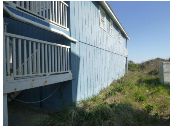
Under Floor Framing & Support: View of exterior finished walls obstructing support pilings
