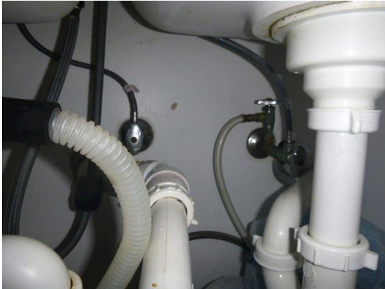
Plumbing: View of plumbing pipes below sinks
