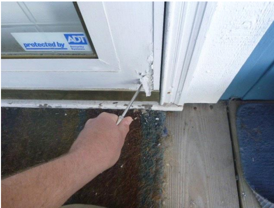
Exterior Doors: View of corrosion present on front storm door
