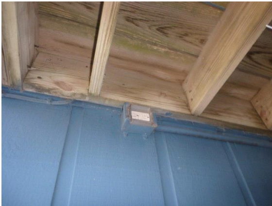
Exterior Surface: View of receptacle with no cover present
