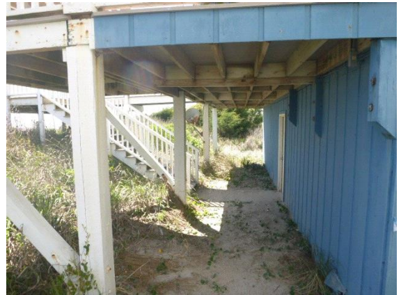
Grading / Drainage: View of rear property with negative slope present
