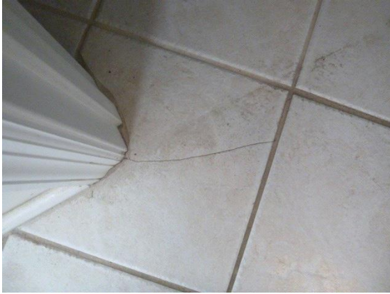
Bathroom #2 - 1st Floor Right: View of cracked bathroom ceramic floor tiles
