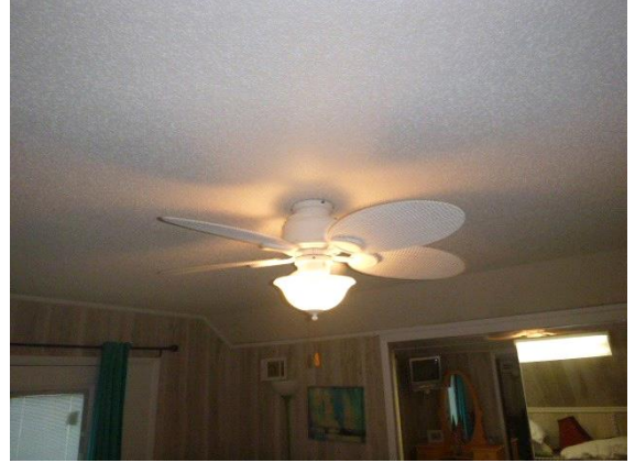
Bedroom #5 - 2nd Floor - Rear : View of noisy bedroom ceiling fan
