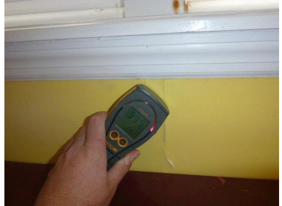
Living Room: View of moisture meter indicating wall stains are wet
