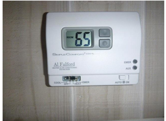
Heating: View of 2nd floor thermostat in heating mode
