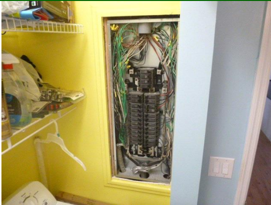
Electrical: View of main electric panel and circuit breaker located in the laundry closet
