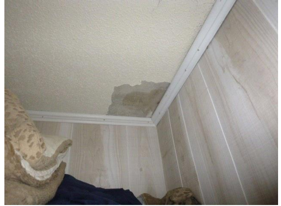
Bedroom #2 - 1st Floor - Front Right : View of water stain located on the bedroom ceiling
