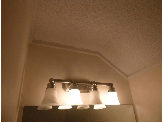
Bathroom #3 - 2nd Floor : View showing defective bathroom light fixture
