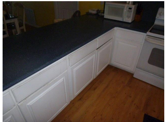
Kitchen: View of kitchen cabinets with no handles present on the doors
