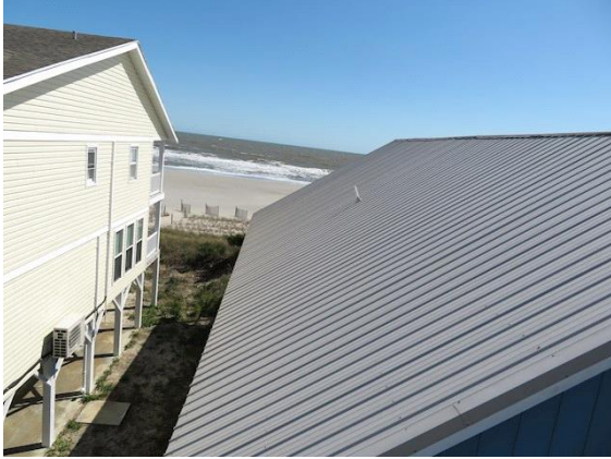
Roofing: Overall view of standing seam metal roof
