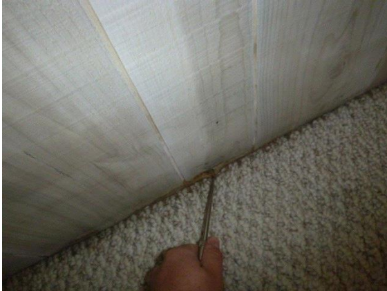
Bedroom #1 - 1st Floor - Front Left : View of one location of soft wall paneling and water staining
