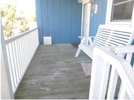
Decks - 1st Floor - Front : Overall view of front 1st floor wood deck
