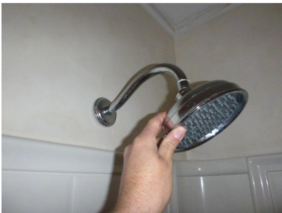
Bathroom #3 - 2nd Floor : View of loose shower faucet
