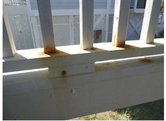
Decks - 1st Floor - Front : View of one location of rusted fasteners on front deck
