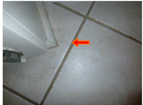
Bathroom #4 -1st Floor Left: View of cracked bathroom ceramic floor tiles
