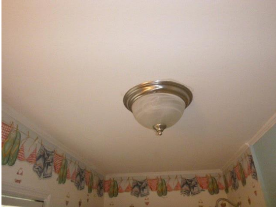
Bathroom #4 -1st Floor Left: View showing defective bathroom light fixture
