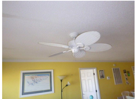
Living Room: View of one location of fan that did not operate
