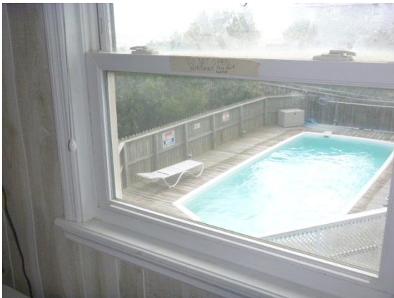
Bedroom #2 - 1st Floor - Front Right : View of window that would not open when using a reasonable amount of force located in the bedroom
