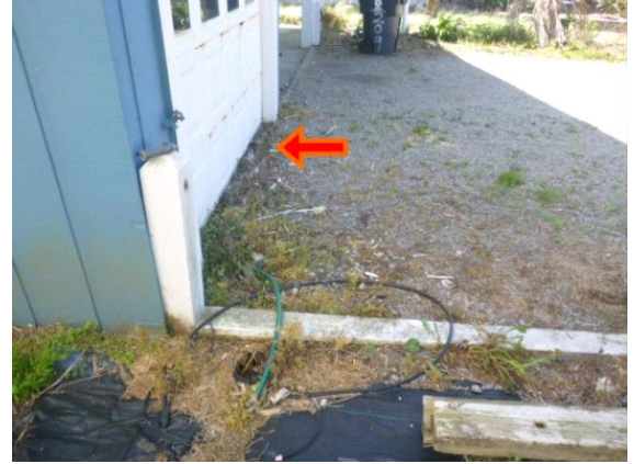
Driveway: View of negative slope in gravel driveway near roll up door
