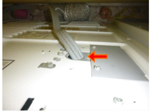
Laundry Facilities: View of missing strain relief connector on the dryer cord
