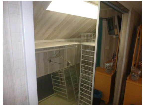
Bedroom #5 - 2nd Floor - Rear : View of one location of missing closet door
