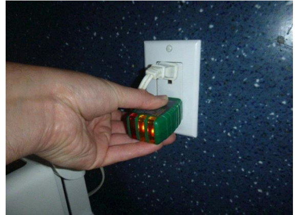
Kitchen: View of one location of kitchen wall receptacle that is not GFCI protected
