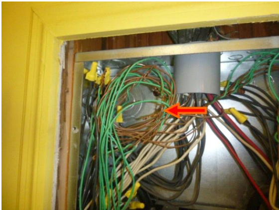
Electrical: View of ground wire connections with no caps or connectors present
