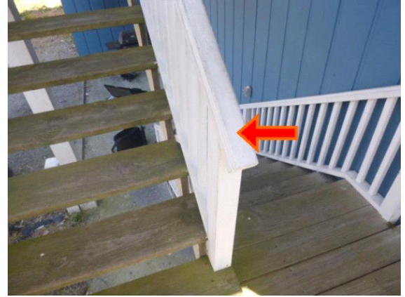
Walks / Steps: View of loose handrail located on the front wood steps
