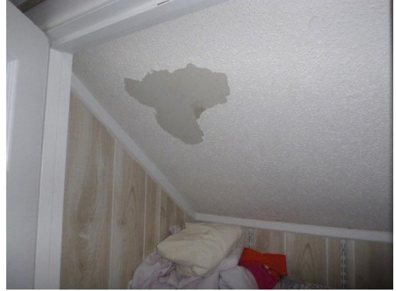
Bedroom #4 - 2nd Floor - Front : View of water stain located on the bedroom ceiling
