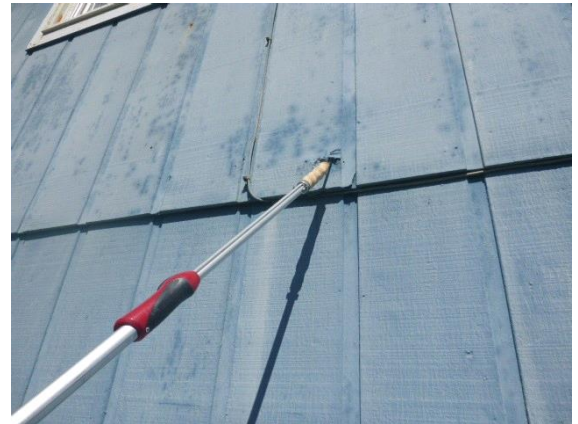
Exterior Surface: View of one location of soft deteriorated wood siding
