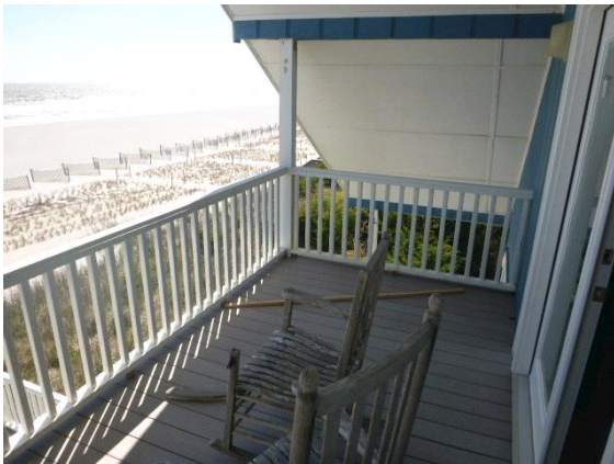
Decks - 2nd Floor - Rear : Overall view of rear wood deck
