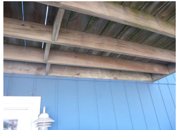
Decks - 2nd Floor - Front : View showing the deck ledger board not bolted to the house
