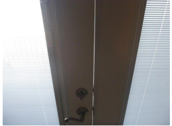
Exterior Doors: View of gap in weather stripping at rear 2nd floor entry door
