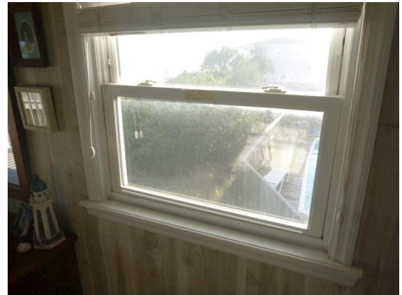
Bedroom #3 - 1st Floor - Rear Right: View of window that would not open when using a reasonable amount of force located in the bedroom
