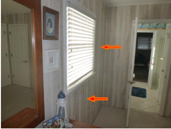
Bedroom #3 - 1st Floor - Rear Right: View of one location of buckled wall paneling
