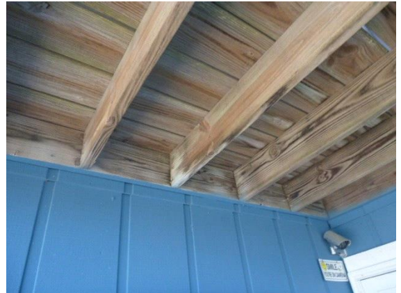
Decks - 1st Floor - Front : View of missing joist hangers or ledger strips at the ends of the floor joists
