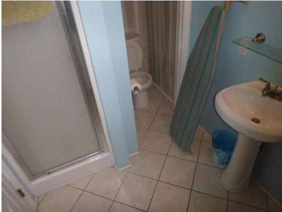
Bathroom #1 -1st Floor Middle : Overall view of bathroom
