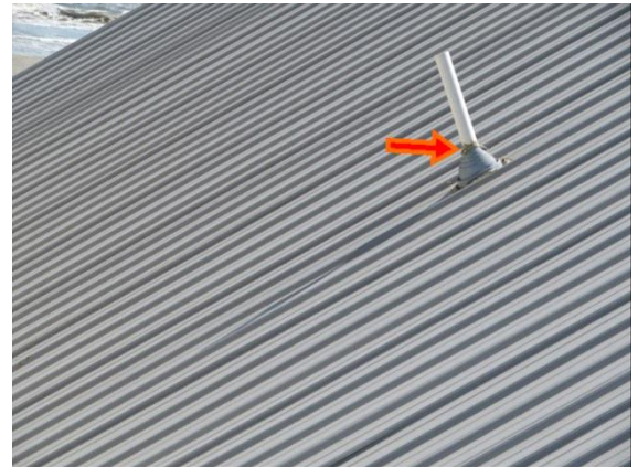
Flashing/Valleys: View of one location of previous repairs to flashings
