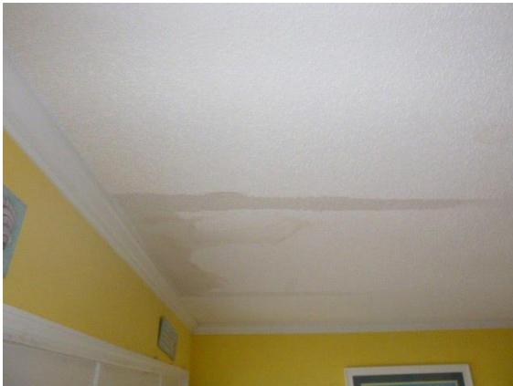
Living Room: View of water stain located on the living room ceiling
