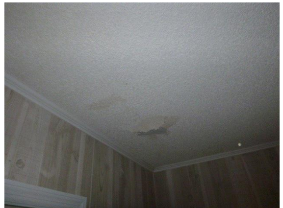
Bedroom #1 - 1st Floor - Front Left : View of one location of water stains present on ceiling
