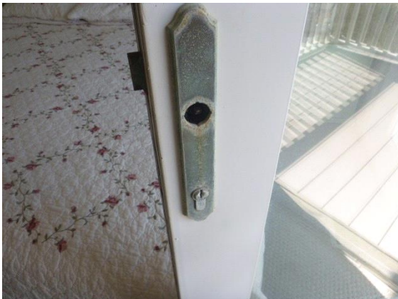
Exterior Doors: View of rear door with binding hardware and handle missing
