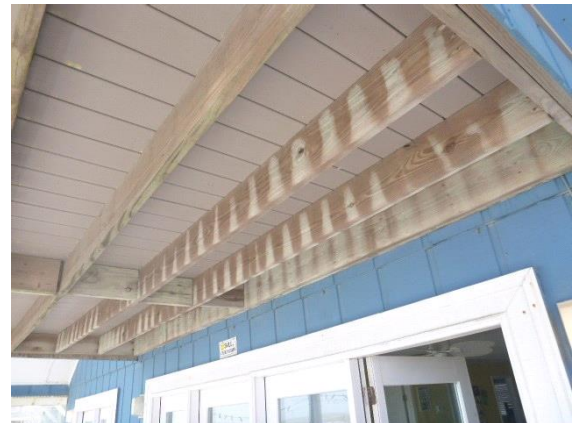
Decks - 2nd Floor - Rear : View showing the deck ledger board is not bolted to the house
