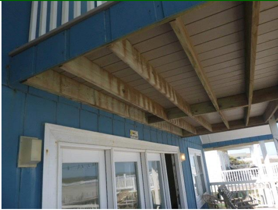
Decks - 2nd Floor - Rear : View of missing joist hangers or ledger strips located at the ends of the floor joists
