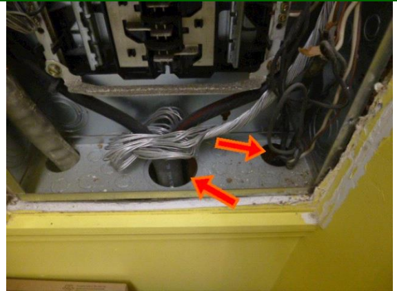
Electrical: View of one location of cables entering the electric panel that do not have the required connectors present
