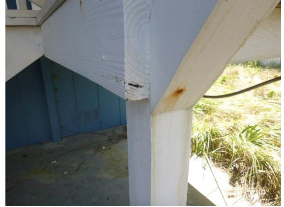
Decks - 2nd Floor - Front : View of one location of rusted fasteners on front decks
