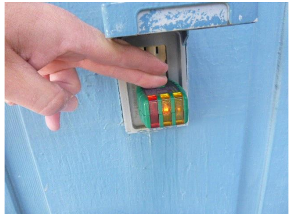
Exterior Surface: View of exterior wall receptacle that is not GFCI protected
