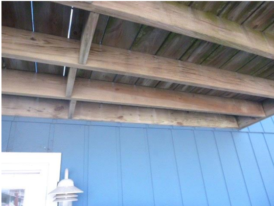
Decks - 1st Floor - Front : View showing the deck ledger board not bolted to the house
