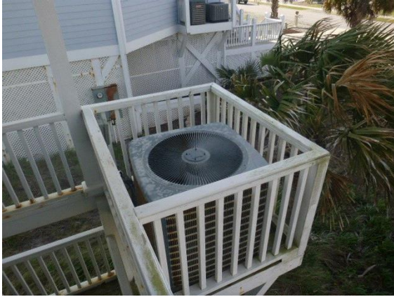
Heating: View of HVAC condenser located on the front of house
