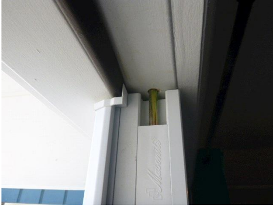
Exterior Doors: View of one location of 2nd floor rear entry door pins that do not fully latch into frame
