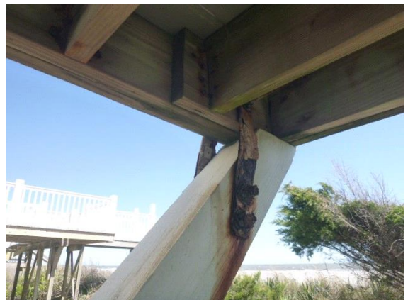
Decks - 1st Floor - Rear : View of one location of rusted fasteners on rear deck
